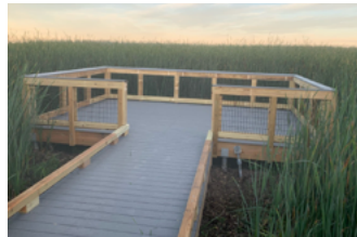
Hellicat Trail Boardwalk Replacement Newburyport, MA US Fish & Wildlife $2,717,000
