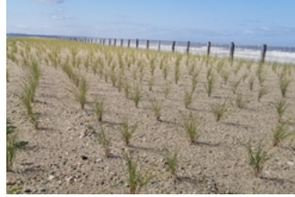
Dune Re-Nourishment Between Crossovers 1 & 2 Duxbury, MA Duxbury Beach Reservation $1,305,731
