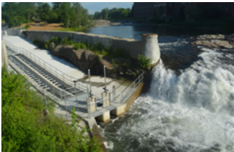
Saccarappa Fish Passage Construction Westbrook, ME Sappi North America $4,479,400
