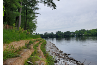
Merrimack River Stabilization Project Chelmsford, MA Town of Chelmsford $2,863,433
