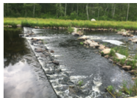
Kenyon Mills Dam Removal and Rock Ramp Fishway Kenyon Mills
