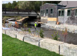
Elm Street Dam Removal and River Restoration Kingston, MA
