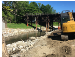
Mill Street Dam Removal and River Restoration Pittsfield, MA
