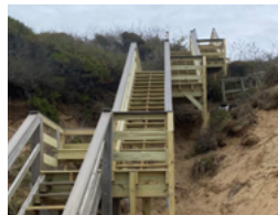
Beach Access Stair Set Truro, MA
