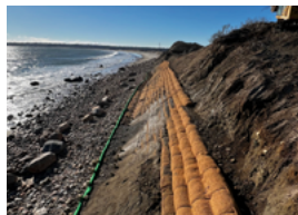
Corn Neck Road Coir Fiber Roll Installation Block Island, RI
